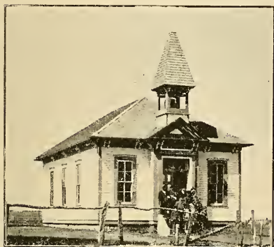
FRAME SCHOOL-HOUSE, Wabaunsee.
