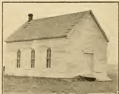
SWEDISH LUTHERAN CHURCH, Mill Creek Township.
