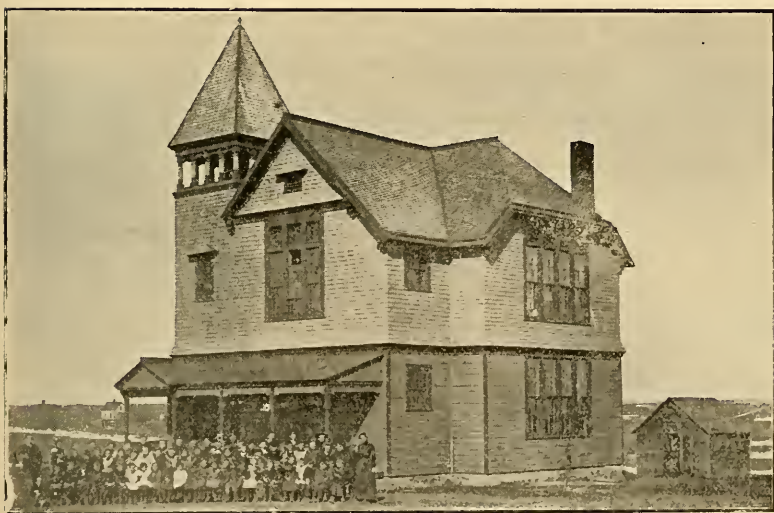
SCHOOL HOUSE. ALTA VISTA.
