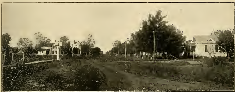
ALMA—LOOKING WEST FROM THE SANTA FE DEPOT.
