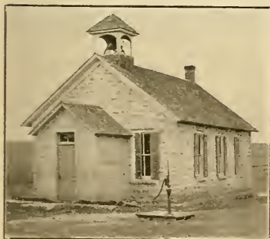
SCHOOL-HOUSE, District No. 45.
