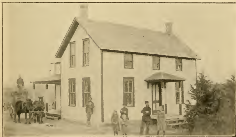
RESIDENCE OF MR. AUGUST HANSEN, near McFarland.
